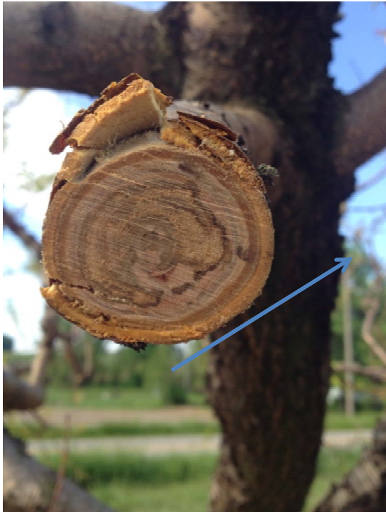
Deterioration of inner wood layers
